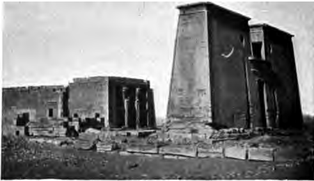
FIG. 11.—Pselkis: Temple and Pylon.
